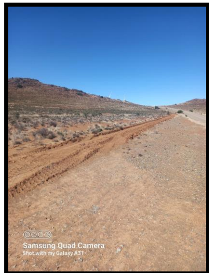
Photo 6: Evidence of erosion remediation along the access road.
